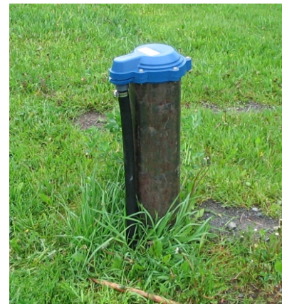
Figure 1. Drilled well water source
